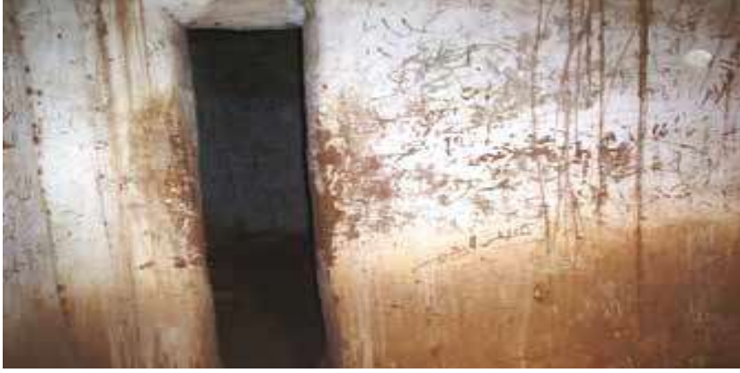
Plate13: The entrance of the small room inside Khalwat El-Sayid el-Hassan.
